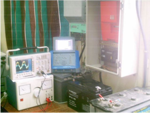
Fig. 5.31 Circuit measurement of battery impedances
